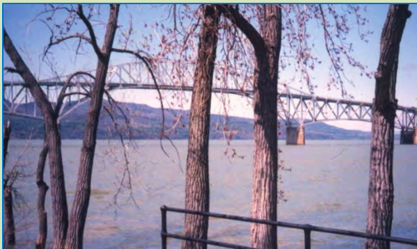
Crown Point Bridge over Lake Champlain from dock at the Crown Point Lighthouse April, 1998
